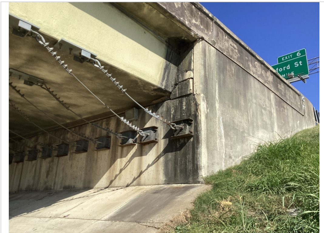
Spall about 2 backwall
