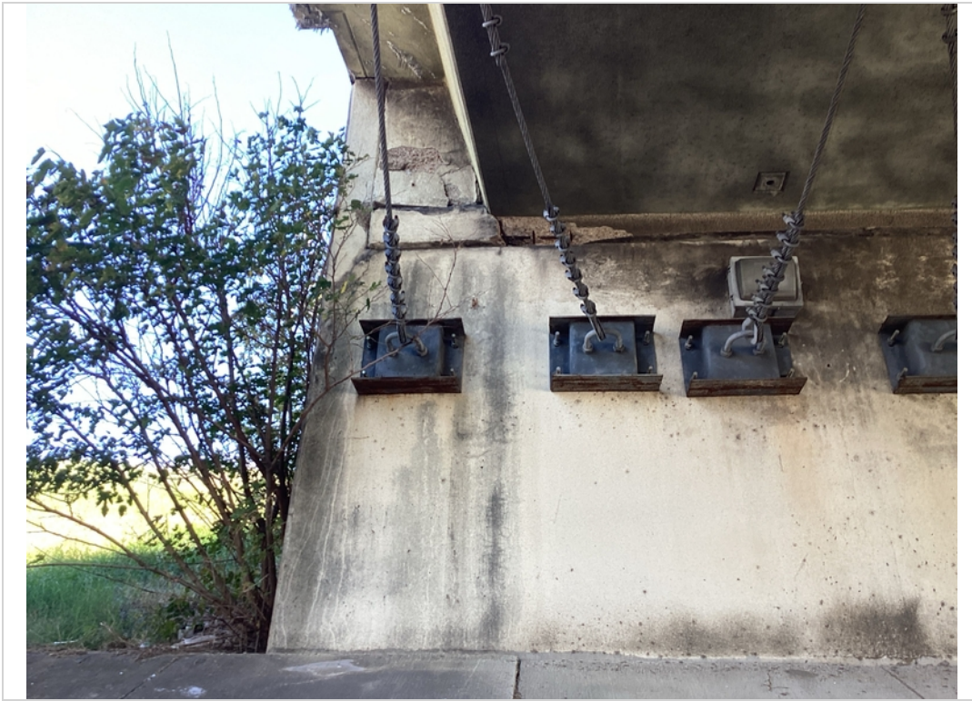
Spall abut 2 back wall
