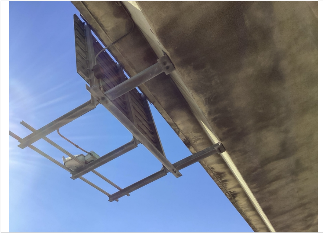
Back of bridge mounted sign
