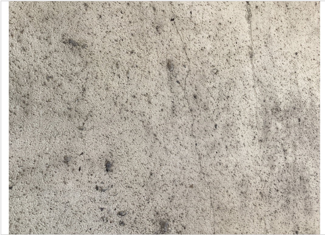
Abutment 1, hairline crack
