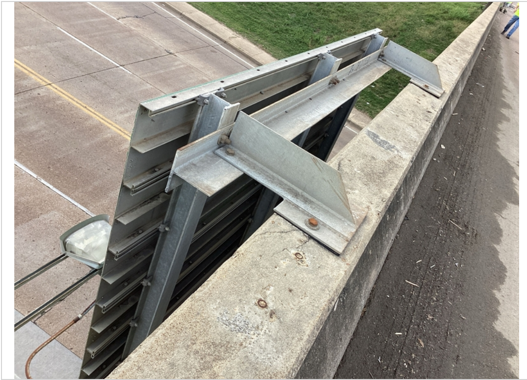
Back of bridge mounted sign
