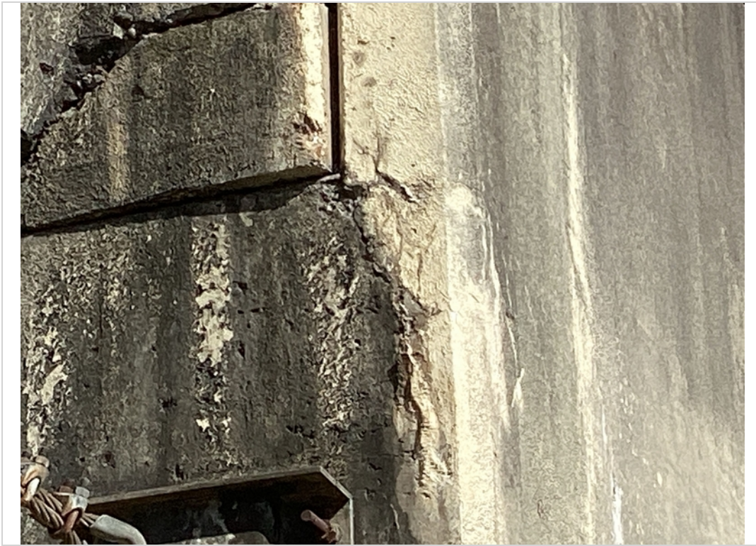
Abutment 2 crack
