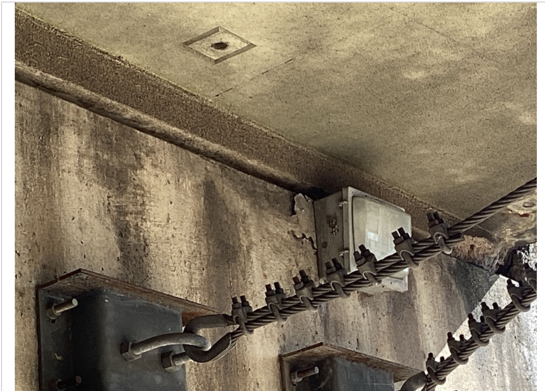
Abutment 2 impending spall
