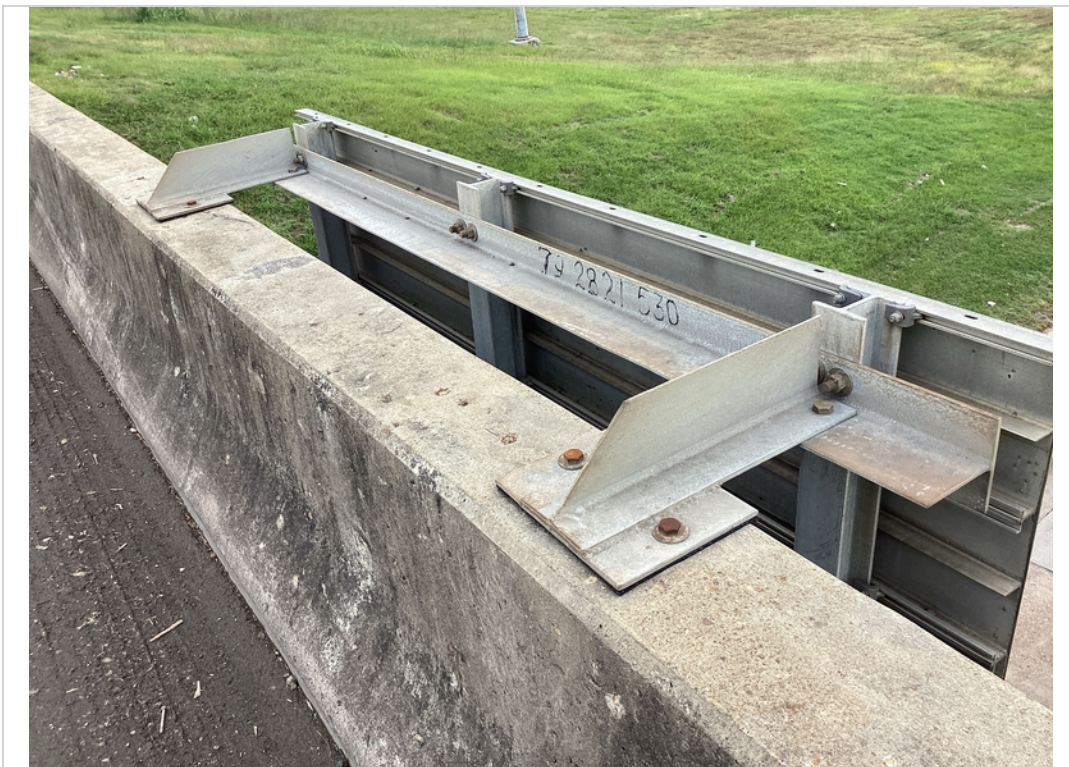
Bridge mounted sign upper connection
